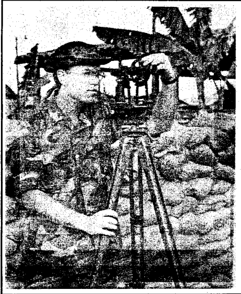
FIRST MISSION — SSGT James P. Bobbit, a site developer, 123d CES, determines elevation at Soto Cano Air Base, Honduras, with a transit. Bobbit was one of fifty-seven members of the 123d Civil Engineering Squadron to deploy to Honduras in the KyANG's first mission as a tactical airlift wing. (Photo by SSGT Jeff Sansbury, 123d TAW)
